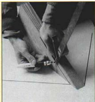
The scrap-block method. Beveling the edges of a valley rafter makes it easier to nail on plywood and drywall. Here, a scrap block cut with the seat cut of the roof pitch is used to find the correct angle.
