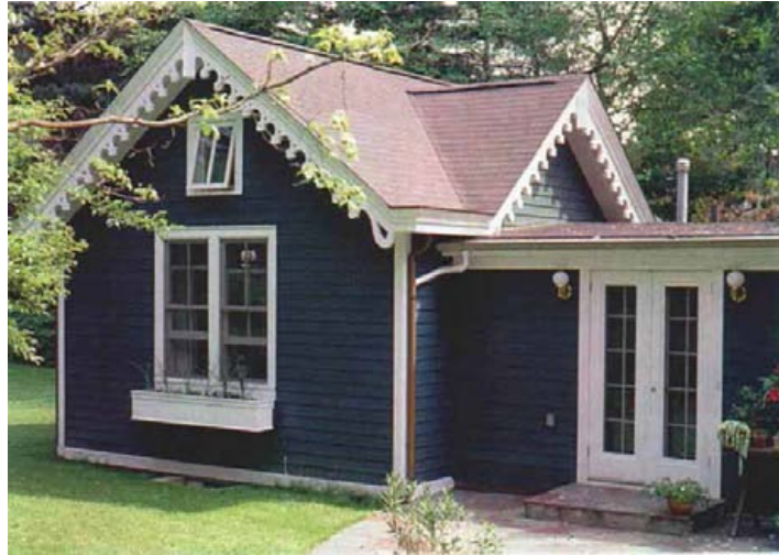
With its cross-gabled roof and decorative vergeboards, this cottage complements the Gothic home to which it's appended. Photo by Kevin Ireton.
